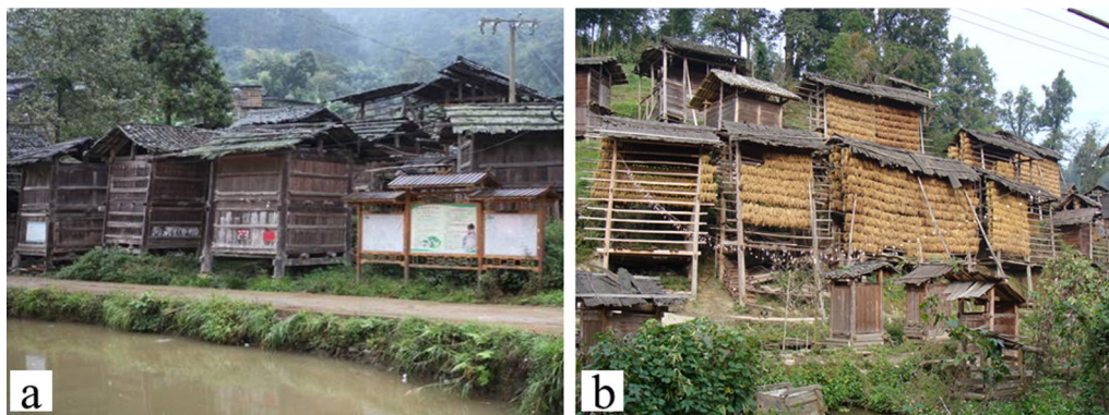
Fig. 4 Granary (a) and heliang (b) were built in a row along the river in Dong village
