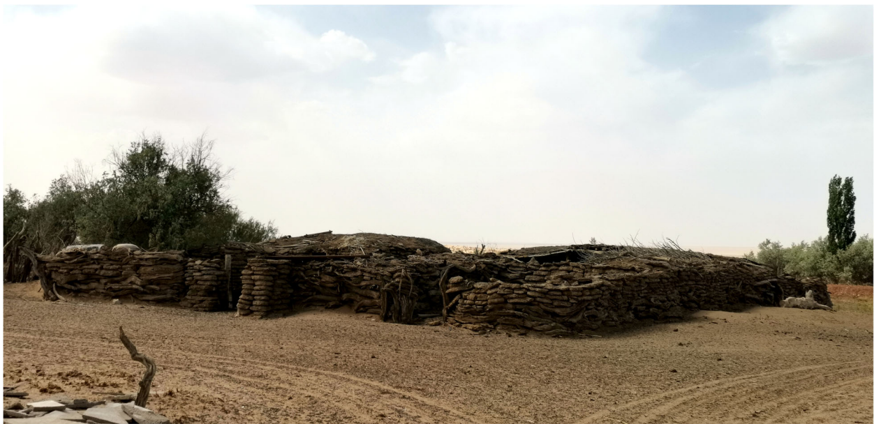
Fig. 11 Stock barns made of Haloxylon ammodendron (C. A. Mey.) Bunge. (Taken by Liu in Ejina)
